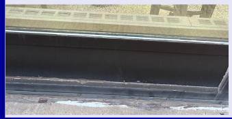
The lintels for the high windows in the pool spectator area are sagging and need replacement before further damage is done to the window and surrounding brick structure. If left unattended, the brick above the header will eventually crack and fall.
